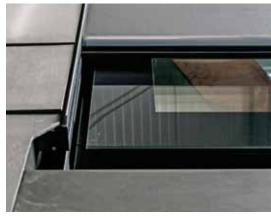
Bottom notch in Eternit panel for lateral drainage.
