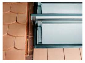
Bottom connection with open louvers and lateral eaves trough.
