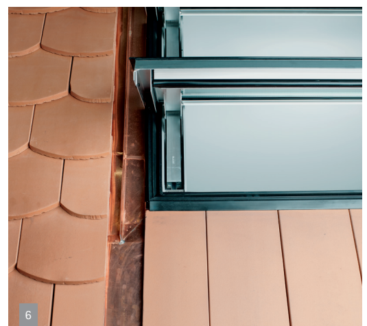
6/9 Bottom interface with open louvers and lateral drip edge.
