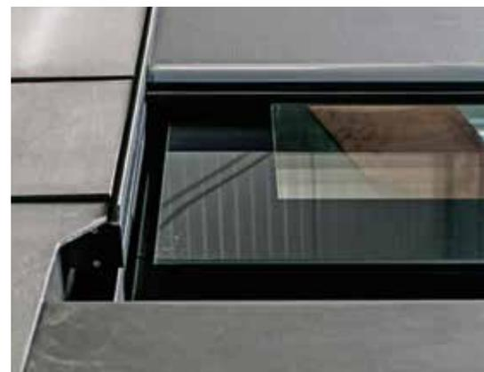
Bottom notch in Eternit panel for lateral drainage.
