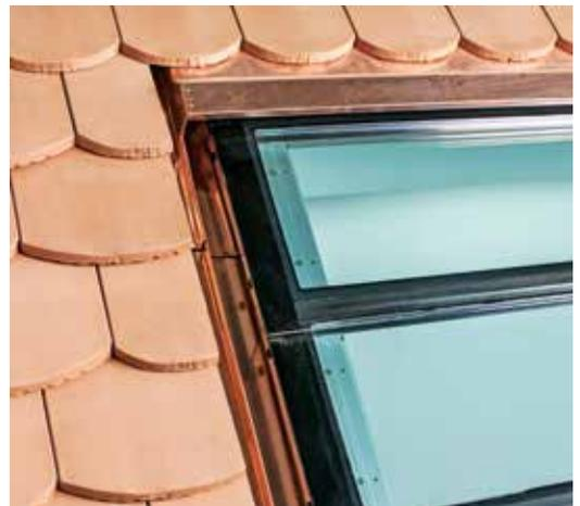
Top connection with tile flushing.
