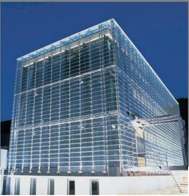
Filigree and attractive. The special method of construction gives our glass lamella a pronounced filigree look. The entire high-grade steel frame construction is reduced to a minimum and harmonises with all building and furnishing styles. It is not without good reason that many designers and architects specify the s: stebler system.
